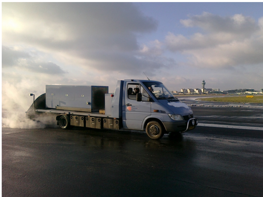
Removing ice layers from a runway
